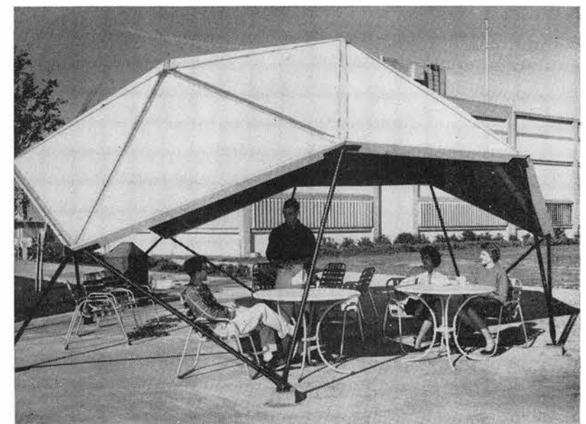
GEODESIC PATIO COVER at Livermore Lab, recently installed in the recreation area south of Bldg. 912, makes possible year 'round use of the patio area during the lunch hour. Relaxing in the shade are, from left, Dale Anderson (8232-2), Dennis Sparger (8232-2), Teresa Pasqual (8232-1), and Sarah Thomsen (8231-1).
